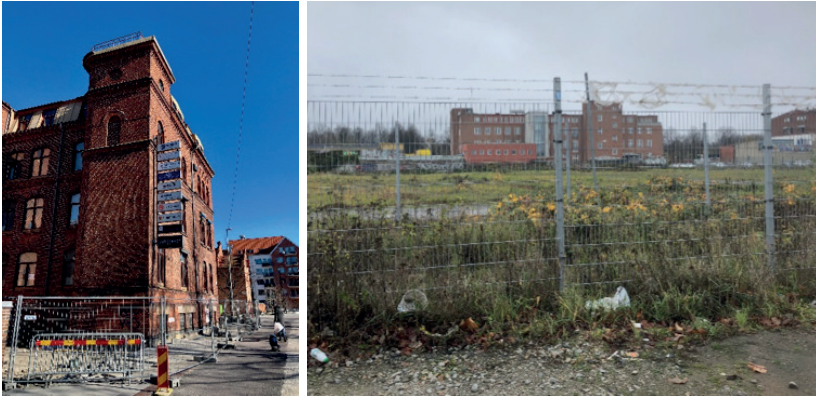
Figure 3 (left): Design ateliers and cultural schools are still housed in this old industrial building
