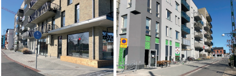
Figure 9 a&b Industrigatan at present when the first block is under construction.
